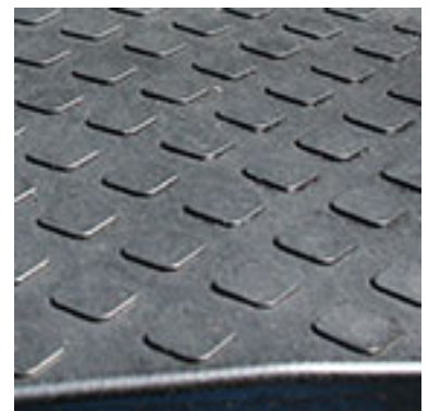
reinforced, curved surface with square imprinting
